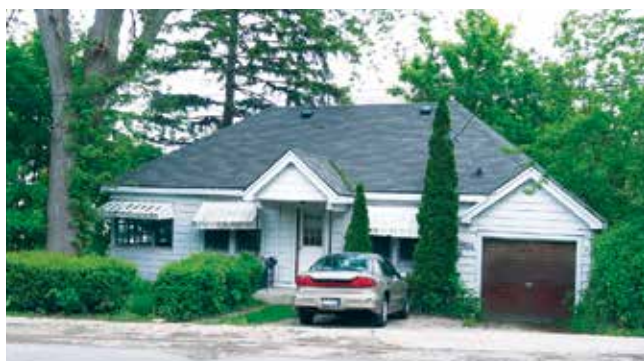
The Mantley house at 44 Lock Street
