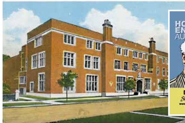
The Downton YMCA was demolished in 1994. A wave of public protest went unheeded by the City. Author Howard Engel (Benny Cooperman Mysteries) chained himself to the doors in protest.
