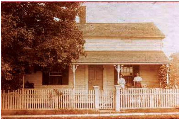
Alexander Muir house, 43 Dalhousie Avenue (Queen Street)
