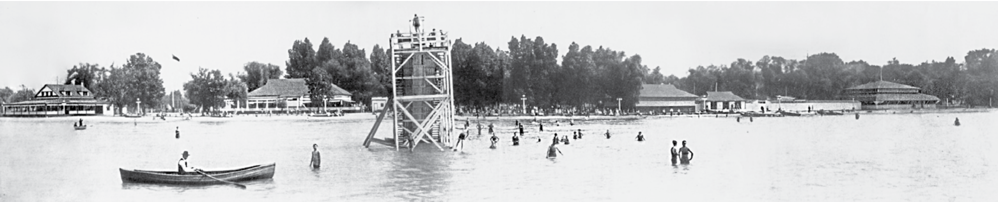
Lakeside Park, 1940: L-R: Restaurant, Dance Pavilion, Bathhouse, Carousel Building
